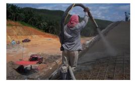
LZ-3A dry mix shotcrete machine/gunning machine is small-sized shotcrete machine for the dry spraying process.LZ-3A shotcrete machine can be used as well for small jobs, such as joint filling, swimming pool, refractory application and extensive slope consolidation work, etc.
